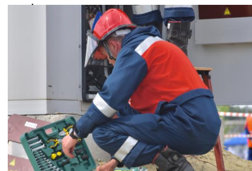
Generator repairs and maintenance
