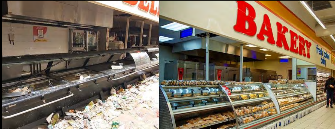
Shoprite Jabulani rebuilt and reopened in just 14 days
