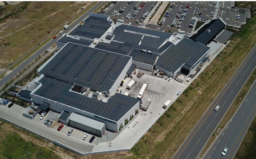
Solar panels installed on the roof of the Sitari Village Centre Mall, Cape Town, Western Cape province.
